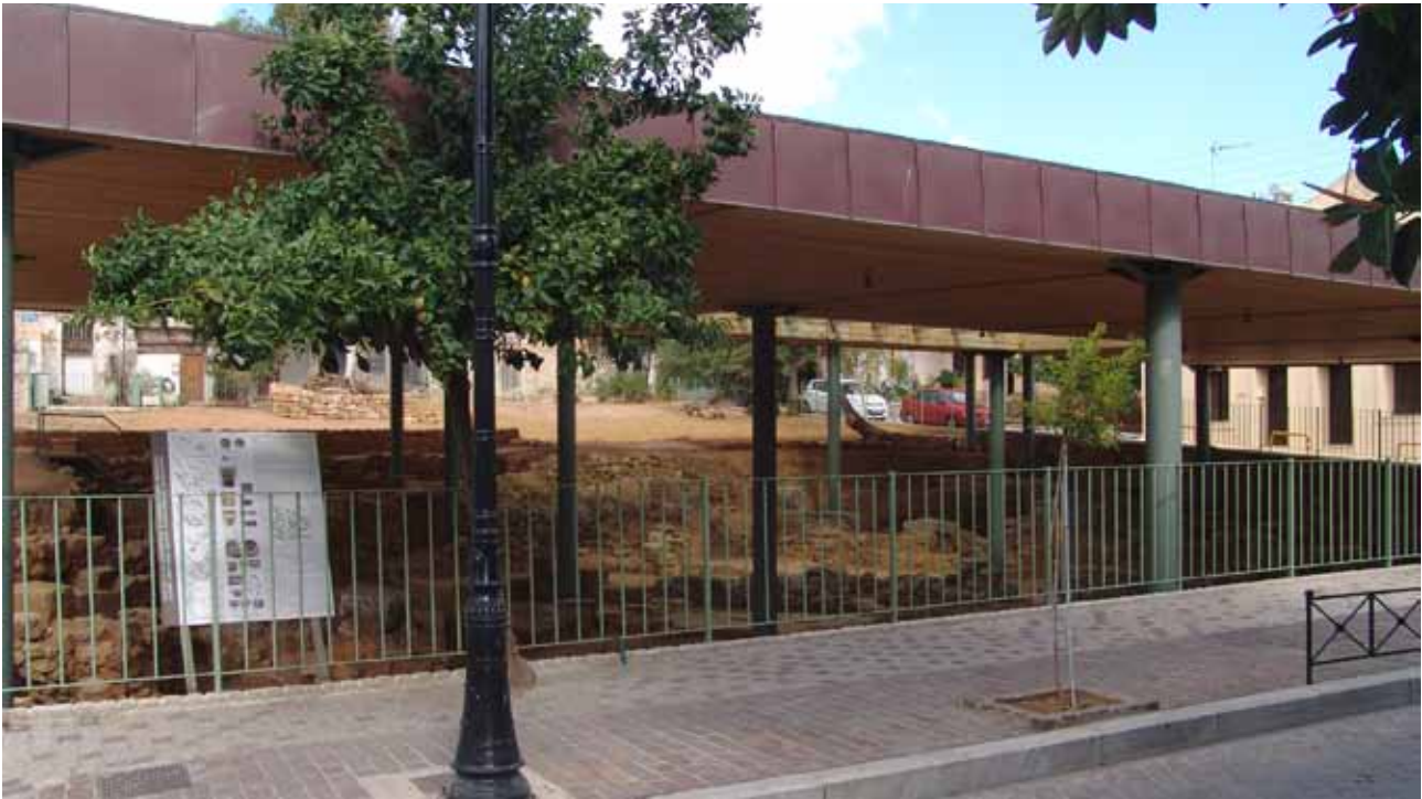
Fig. 5. View over the Ag. Aikaterini Square. The excavated area (backfilled) is in the centre of the photograph outside the protective roof. Facing north. © GSDE 2010.
